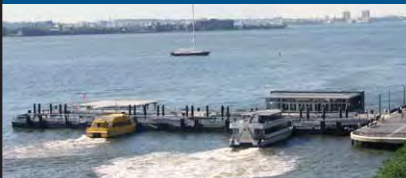
Heliport & Ferry Service
